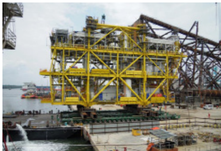
Load-out of two compression modules (1750 Ts + 1865 Ts) for Shell / Petronas Malaysia
