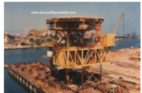
Load-out of 2x700 tons Offshore desk at Hindustan Shipyard in Visakapatnam, India
